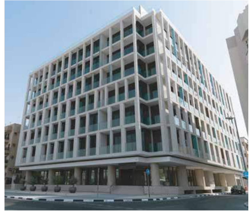
Lootah Building - Al Hamriya-Dubai Client - Lootah Family
