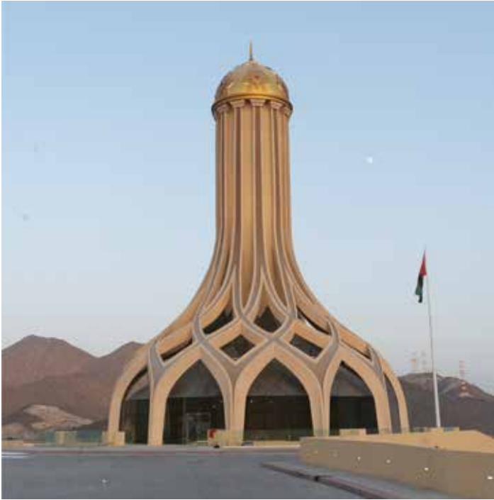
Monument Center - Khorffakan-Sharjah Client - Sharjah Govt
