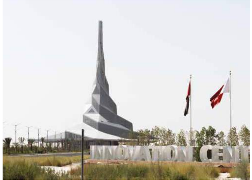
Solar Innovation Tower -AL Qudra-Dubai Client - Dewa
